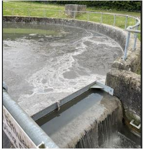
Storm and final effluent have a combined discharge point on site, which causes the FE to backup when site is going to storm, this in turn submerges the UMON4 - as see while on site. Is there a plan to separate these flows out?
