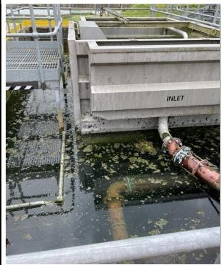
This is being pumped into the returns well. The backwash on the TT cloth media also goes to the returns well. However when the returns well is full, the pipe to the TT plant back ups and appears to start building out of the ground.
