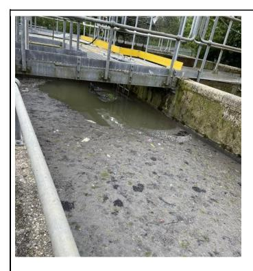
6. FST's 8 FST's on site. Number 5-8 have different media and are clear and free of moss and grass. Number 1-4 need herbicide dosing and filter arms on number 4 needs cleaning.
