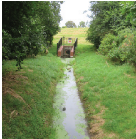
● Flow from Markyate Cell, Aug 2024
