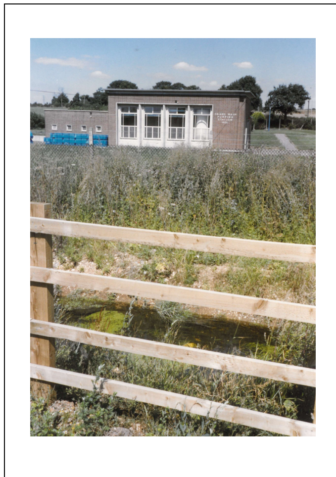
Friars Wash Pumping Station, River Ver, August 1994
