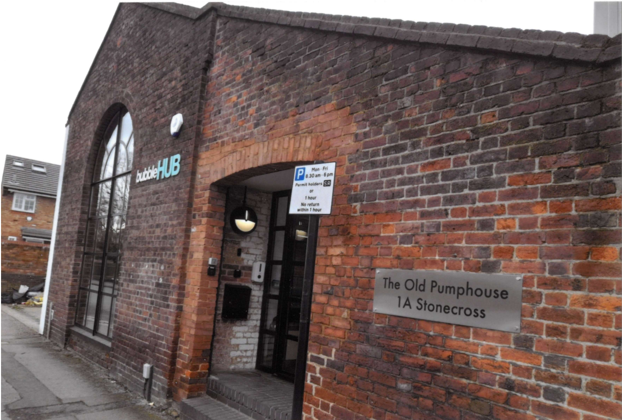
The Old Pumphouse, Stonecross
