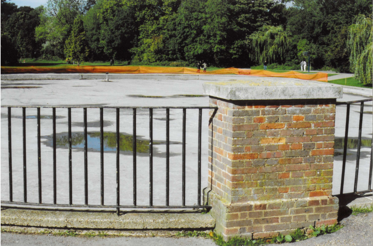
Top/Settling Lake, Verulamium Park, drained and desilted, dry Summer/Autumn (2 nd October 2005)
