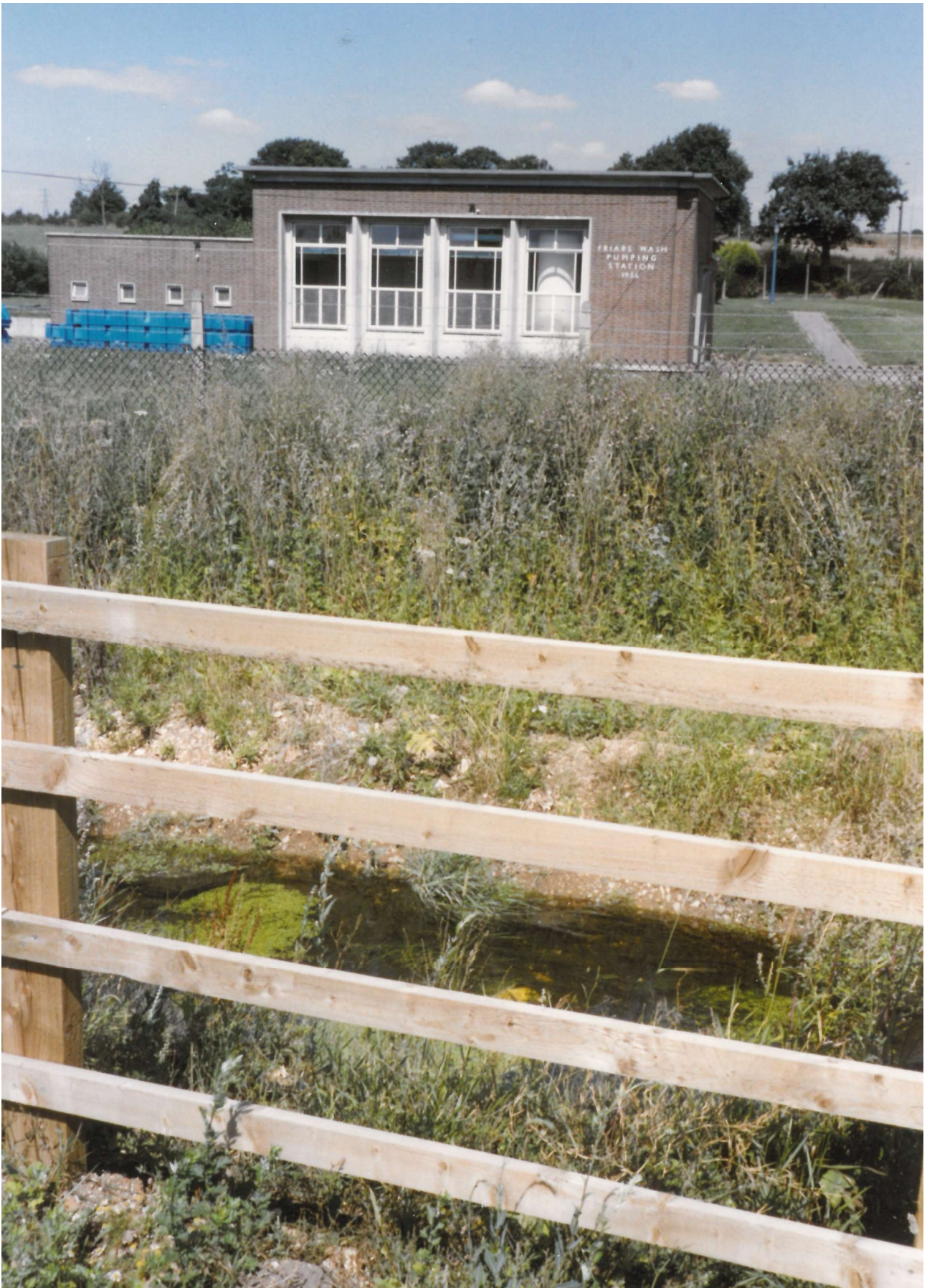
Friars Wash Pumping Station, River Ver, August 1994
