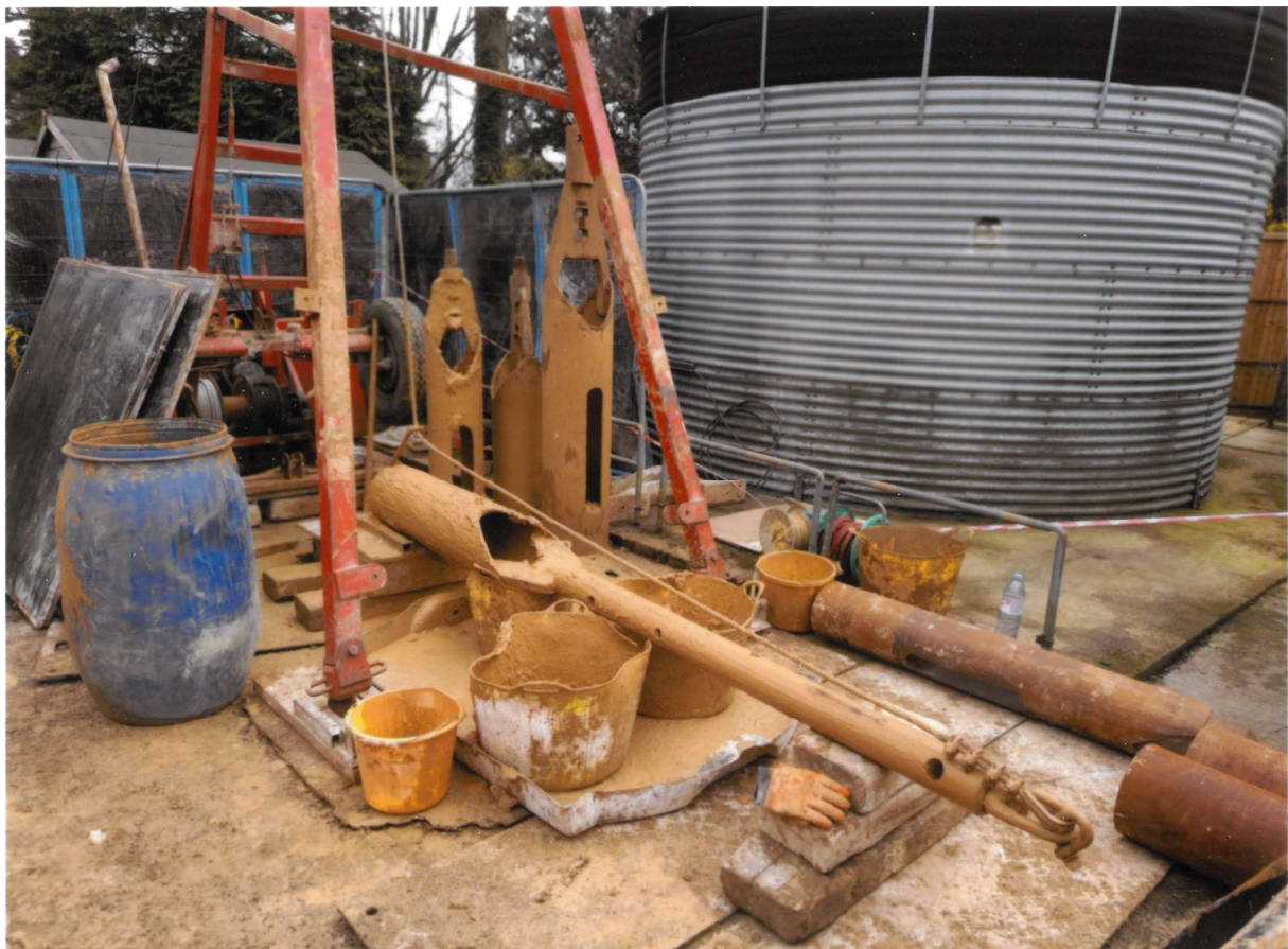
Sinking of a modern borehole/well in the 21 st century, near St Albans
