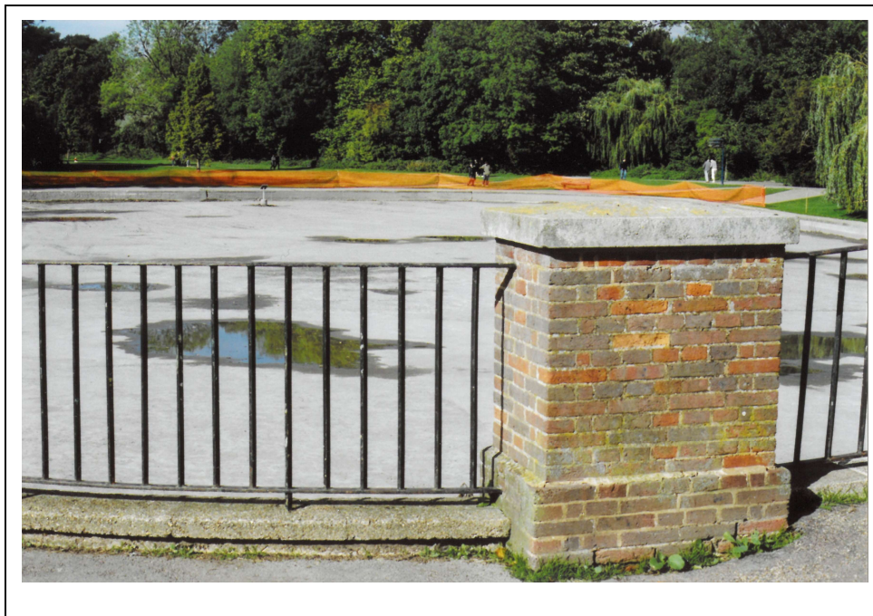
Top/Settling Lake, Verulamium Park, drained and desilted, dry Summer/Autumn (2 nd October 2005)
