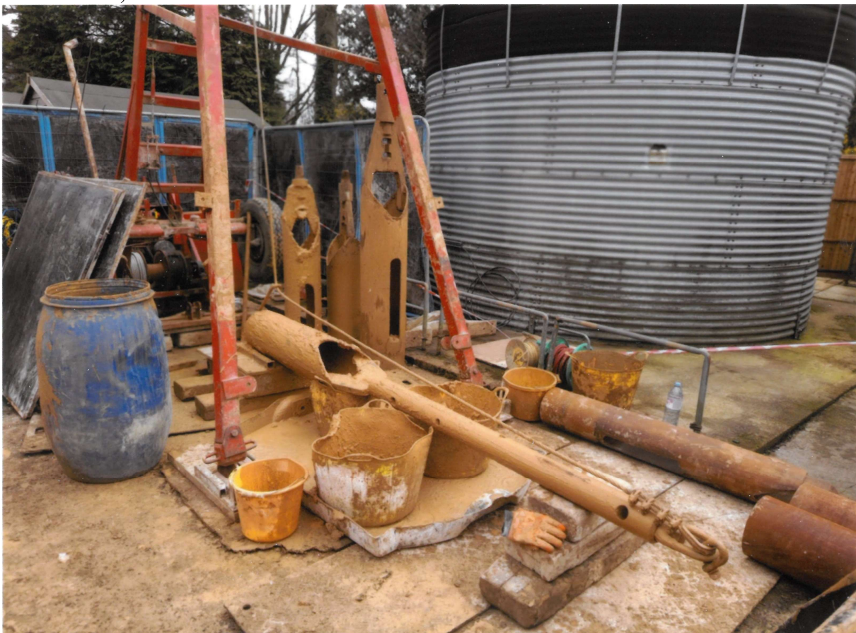
Sinking of a modern borehole/well in the 21 st century, near St Albans
